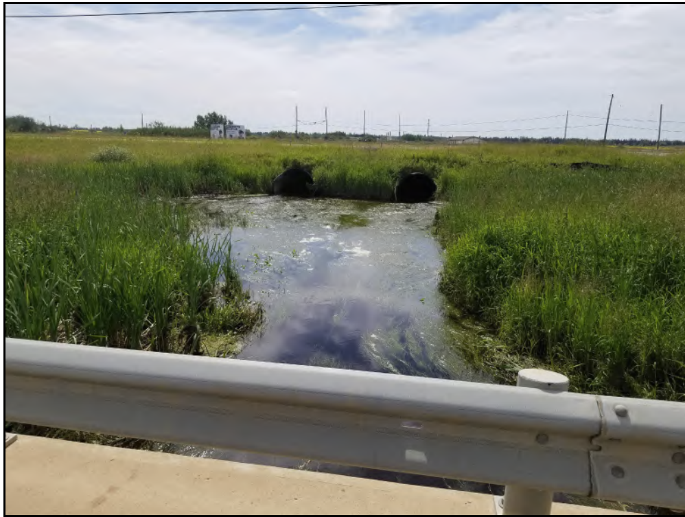
Photograph 3: Facing south from the bridge location, along Horsehill Creek. The river can be seen entering 2 culverts to allow drainage below Highway 15.
