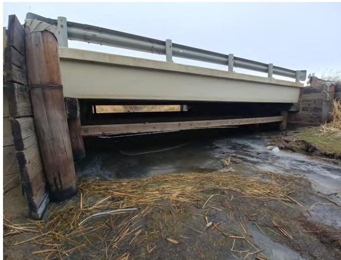
Plate 1.1. Horsehills Road over Horsehills Creek (B130) with single span girder supported by wooden pile abutments (27 October 2020).
