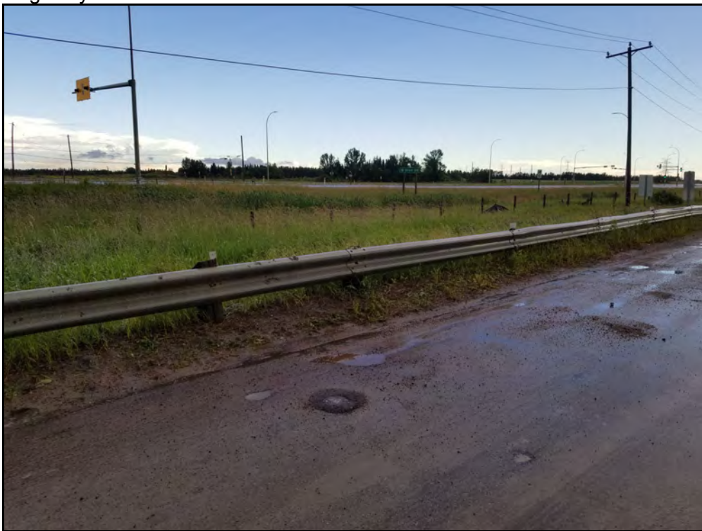
Photograph 4: Completed borehole with flush mounted well protector installed at the surface.
