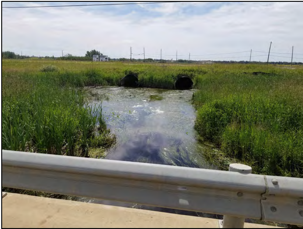
Photograph 3: Facing south from the bridge location, along Horsehill Creek. The creek can be seen entering 2 culverts to allow drainage below Highway 15.
