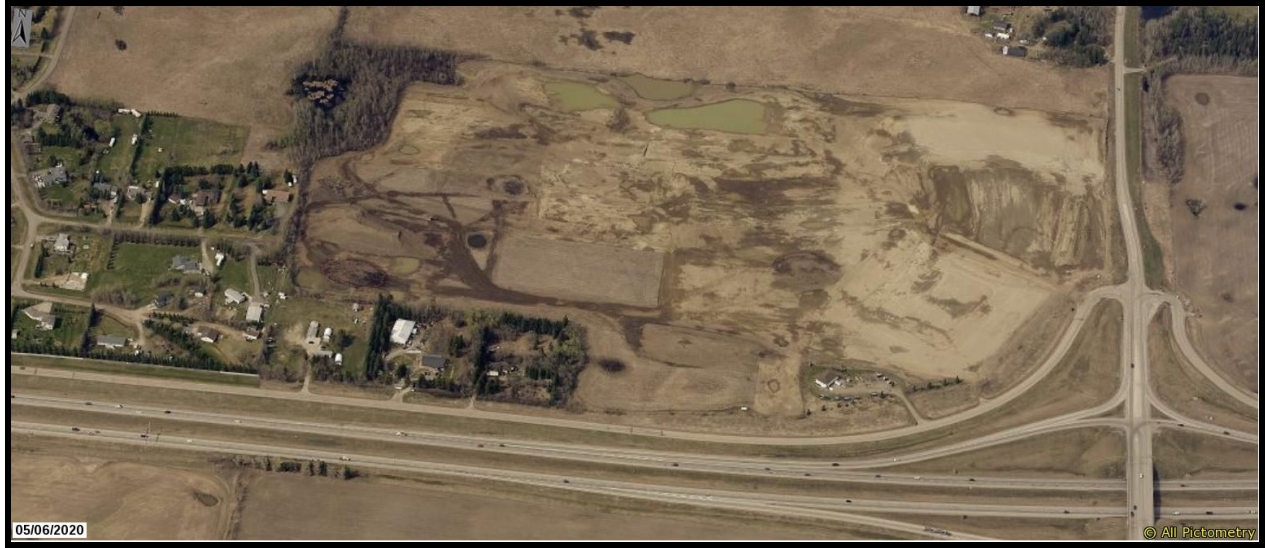
AERIAL VIEW OF SITE LOOKING TO THE NORTH
