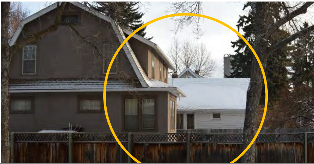
EXISTING INTERFACE WITH ADJACENT HOUSE
