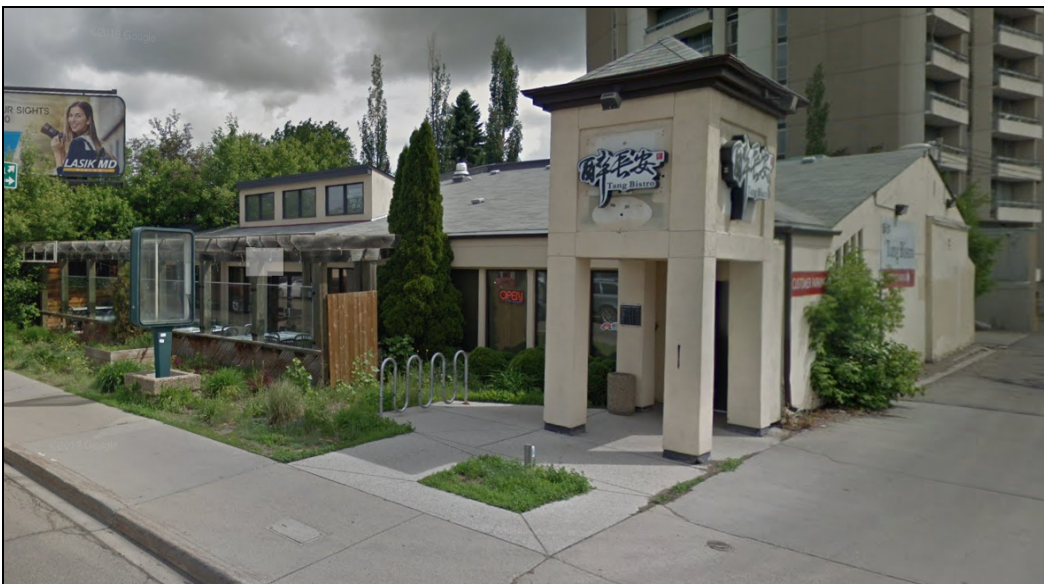
VIEW OF 109 STREET NW SITE LOOKING NORTHEAST
